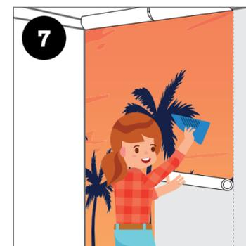
Using a wallpapering tool, gently smooth out any bubbles. Apply adhesive to the wall to prepare it for the next strip. Carefully align it with the first strip, making sure there are no visible seams.
